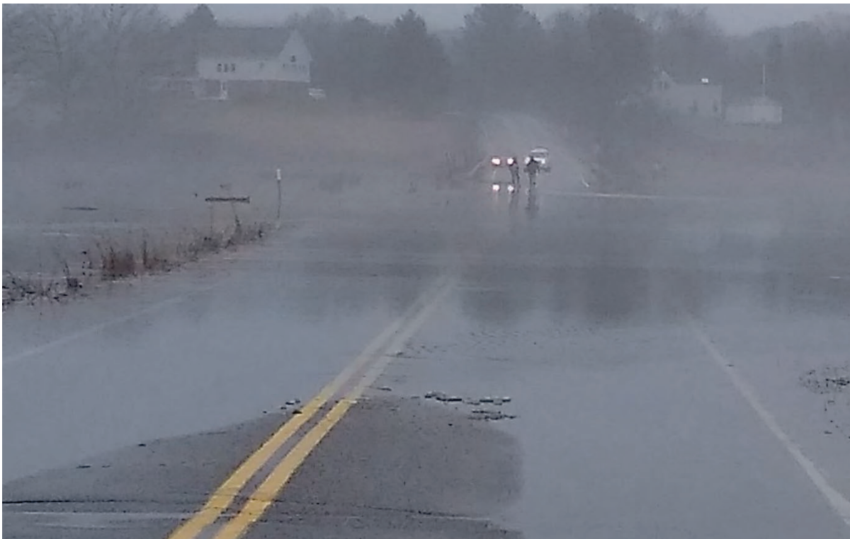
Sawyer Road Crossing Overtopping During High Tide on 12/14/2019 (Photo Credit: Casco Bay Estuary Partnership)
